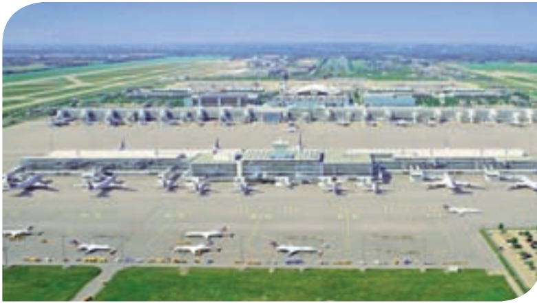
The satellite building in front of Terminal 2 in Munich will make the needs-oriented capacity increase a reality when the summer timetable 2015 comes into effect.
