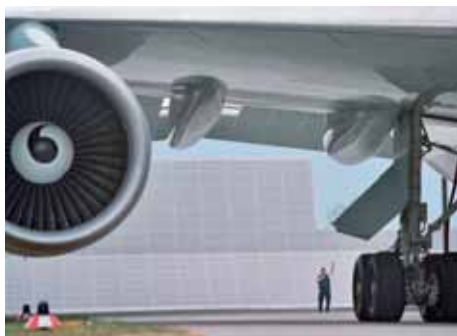
A Lufthansa Boeing 747-400 being towed into the noise protection hangar in Hamburg for a run-up.
